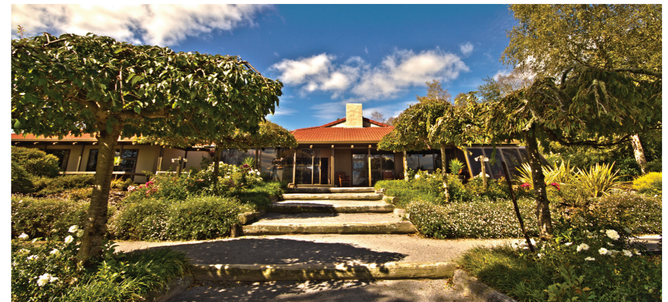
THE RIVER LODGE - KOINONIA HOUSE MINISTRY HEADQUARTERS - REPOROA, NEW ZEALAND
